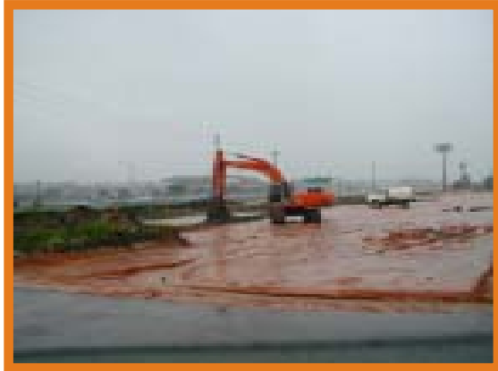
Commercial construction site in the Dog River watershed with minimal soil erosion control
