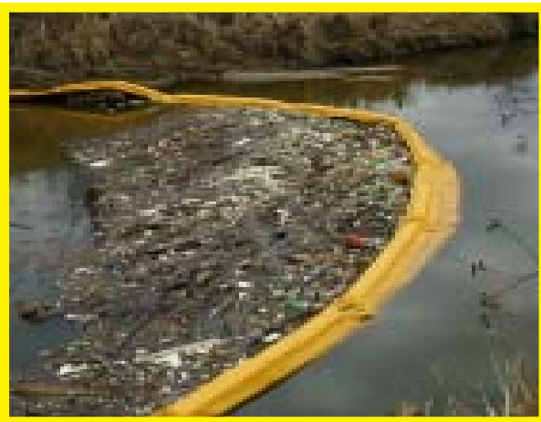
A sediment curtain on Moore Creek catches more litter than silt
